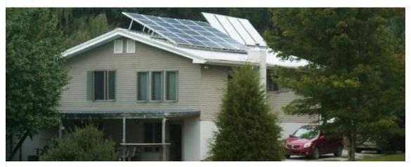
A WORK IN PROGRESS. The PV panels and flat plate collectors on the roof have been raised from their original flush position to better access the winter sun. In the future, David Bolt plans to re-install evacuated tube collectors (that the flat plate devices replaced), in addition to what's on the roof now, to provide space heating for the home.
