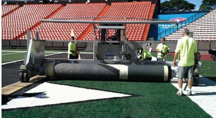
The UBU Sports synthetic turf system has three end zone configurations called **Removable Active Panels or R.A.P. System.** The R.A.P. System allows the end zones at MetLife Stadium to be changed from NY Jets to NY Giants in less than 12 hours. Aloha Stadium, home of the NFL Pro Bowl, was the first stadium to install the UBU Sports R.A.P. System.
