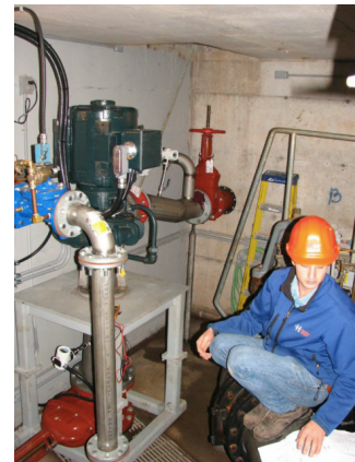
Vertically installed Halifax Water Flow-to-Wire 32 kilowatt system is only 33 inches tall.
