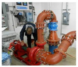
In a pilot installation, SEMS were tested in the water distribution center of the North Wales Water Authority (NWWA), which serves more than 25,000 people in 11 communities in northern Philadelphia. Based on flows of 1,400 gallons of water per minute and a 23 pound per square inch of pressure within the NWWA water transfer station, the system expects to generate 12 kilowatts of electricity, or the equivalent of \$7,500 per year in electricity generated (i.e., not purchased from outside sources).
