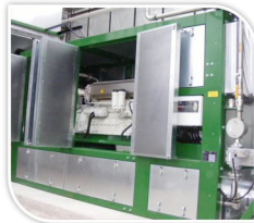
Sewage Gas CHP
