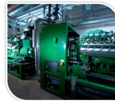
Natural Gas CHP
