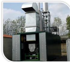
Coalmine Gas CHP
