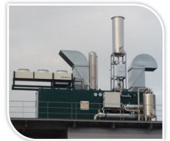
Specialty Gas CHP
