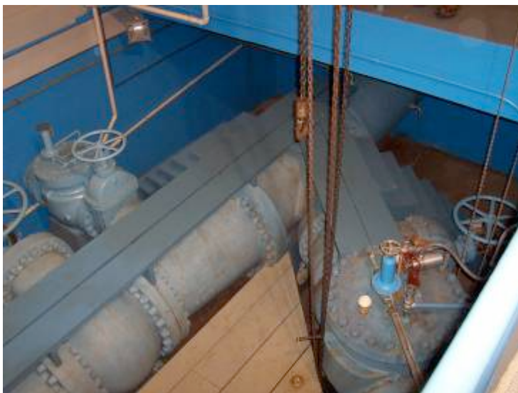
The Hovertown Transfer Vault will be reviewed by Rentricity
