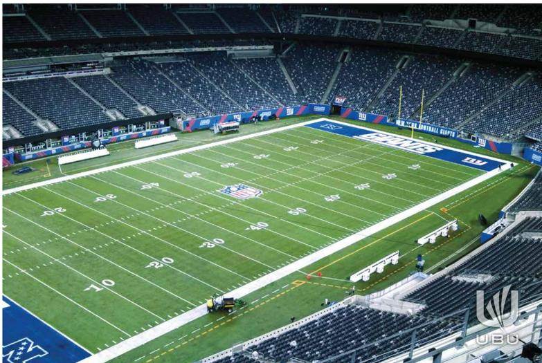
Mark Hill, Director of Quality Assurance for UBU Sports, said, "We finished installing the UBU Speed S5-M synthetic turf system at MetLife Stadium this summer. It features our Removable Active Panel System, which allows us to swap the Jets' and Giants' end zones in less than 12 hours."
