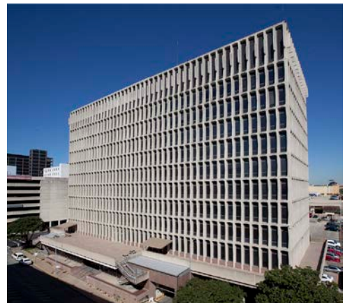
AFG Group will provide Construction Management and Move Coordination for major alterations to the J.J. Pickle Federal Building in Austin, TX.
