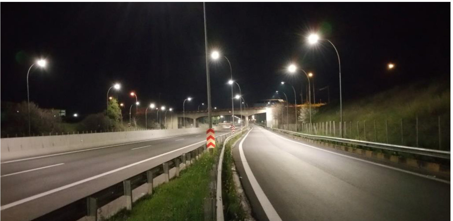
LED Retrofits and LED Fixtures
