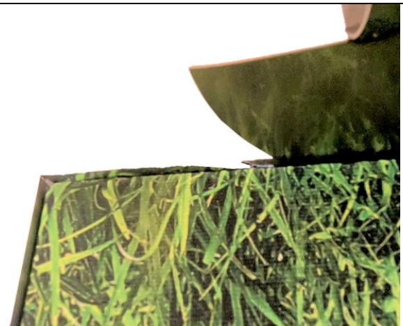
Pushing the visible remaining textile in the groove with the tensor.
