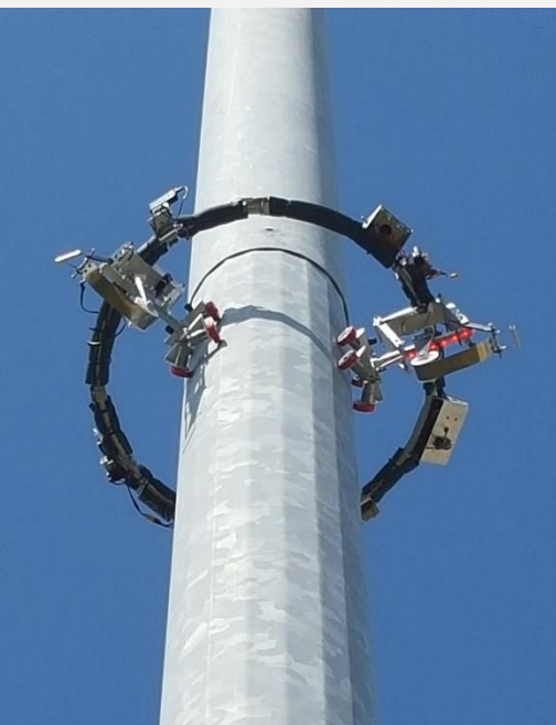
PoleScan™'s repair service robotically sands down rust spots, paints & repairs the high mast light pole.
