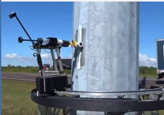
PoleScan™'s repair service robotically sands down rust spots, paints & repairs the high mast light pole.
