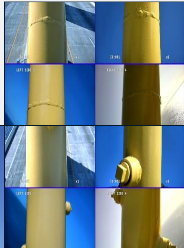
Detail of Grout Ports
