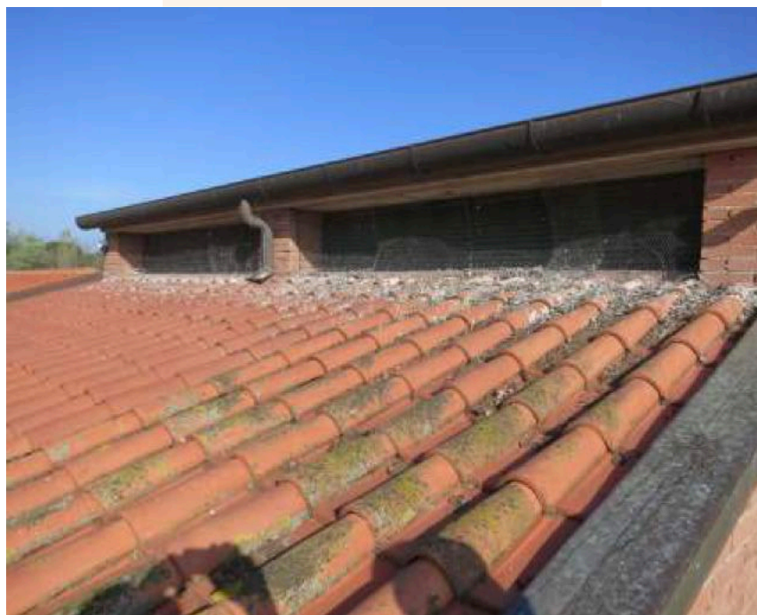
Figure 1. South roof prior to cleaning and treatment.
